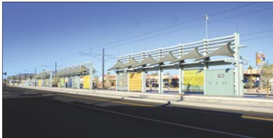
Businesses along the Northwest Extension Phase II that have been impacted by light rail construction can apply for up to $9,000 in financial assistance (a section of Phase I is pictured; photo courtesy of Valley Metro).
