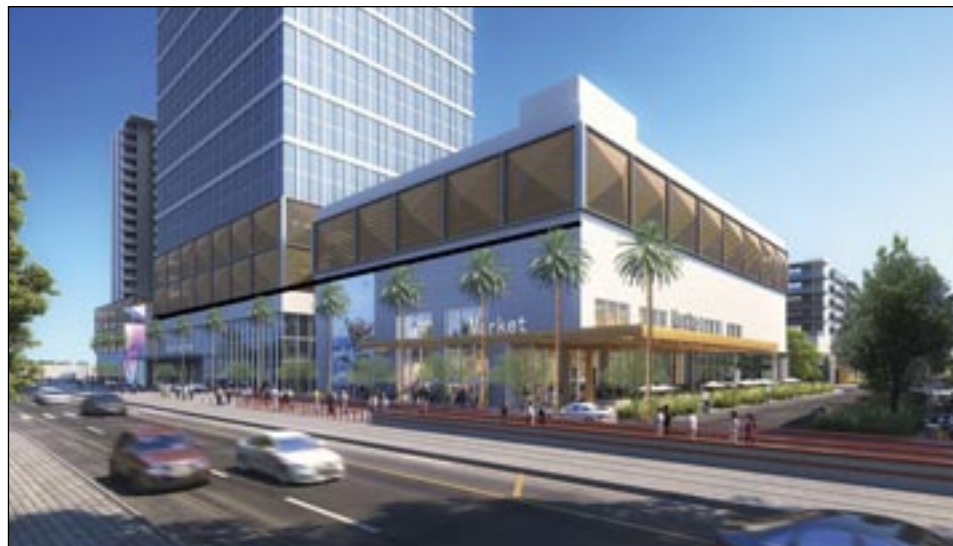
After neighbor input received at an Aug. 21 meeting, the developer of The Central Park will bring the proposed grocery store to a more prominent place along Central Avenue at Monterosa Street (rendering courtesy of Pivotal Group).
