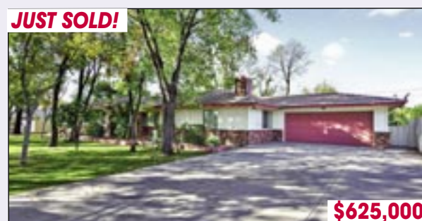
7730 N. 7th Avenue Large prime lot with no HOA
