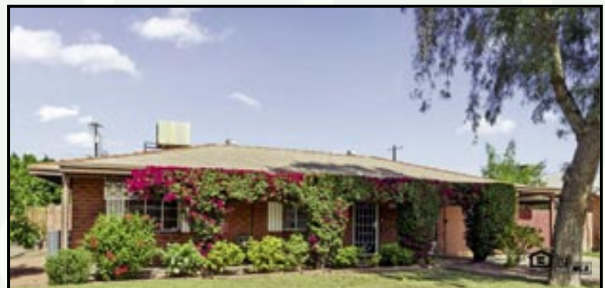
1936 W Clarendon Ave, 85015 Under Contract
