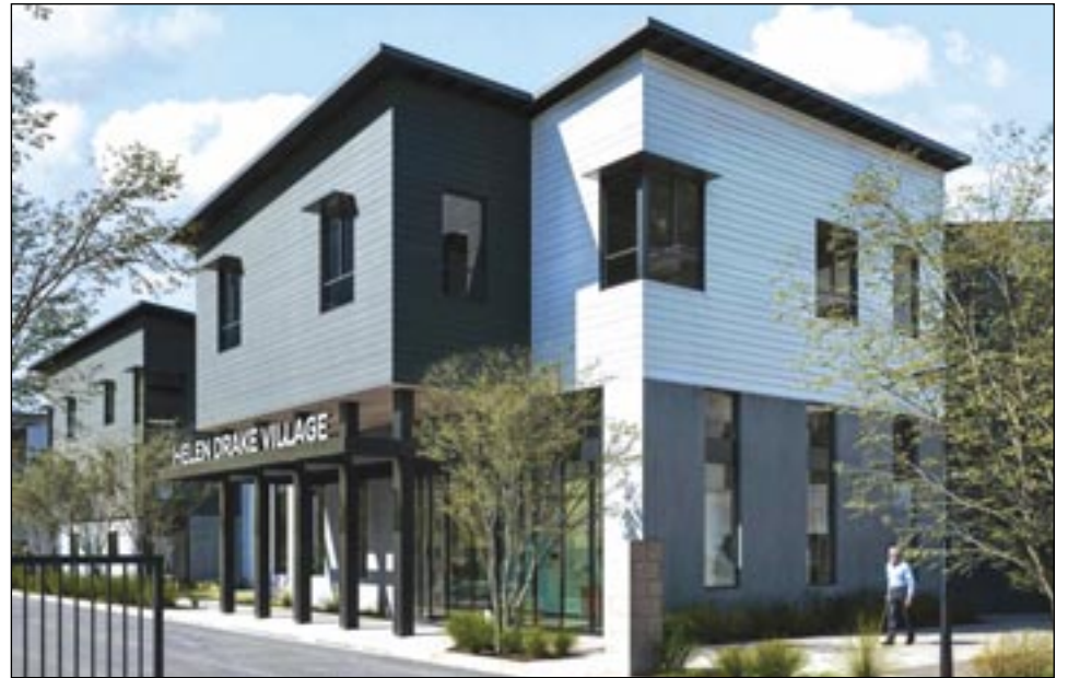
Construction on the Helen Drake Village, a new affordable housing community that will bring 80 rental homes to Phoenix seniors, is anticipated to be completed in 2027 (photo courtesy of City of Phoenix Housing Department).
