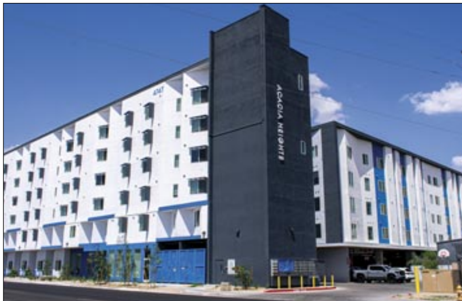
Located just south of Camelback Road on 7th Avenue, affordable housing complex Acacia Heights in May celebrated the completion of its third and final phase, which brings 68 more units to the site (submitted photo).
