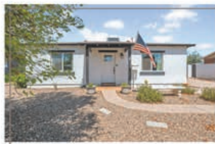
4247 N 4TH Ave | Phoenix, AZ 85013 Stunning Home in Melrose District of DTPHX
